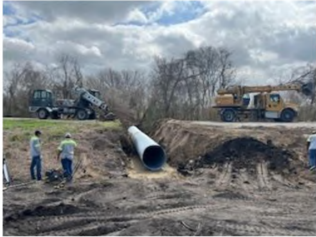
Figure 24 - Bosse Road Culvert Installation 3/5/2026
