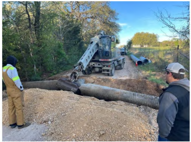
Figure 25 – Dannheim Road Culvert Replacement 3/17/2026
