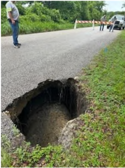
Figure 23 - Quebe Road Culvert Failure 6/12/2025
