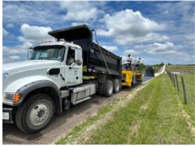
Figure 15 – Whitman Road Chip Seal Application 5/11/2026
