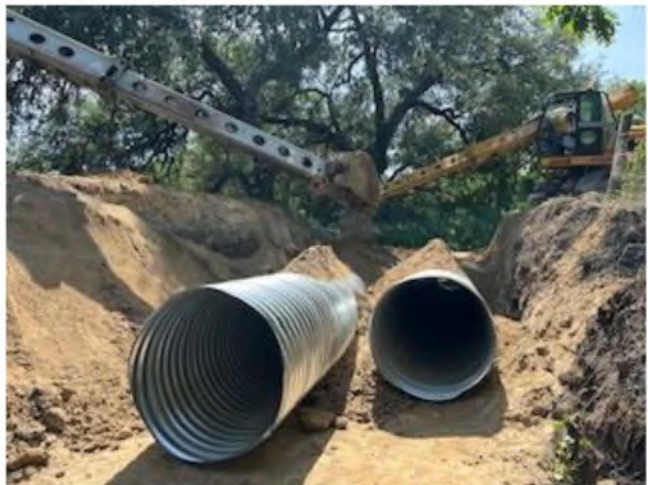
Figure 22 - Quebe Road Culvert Replacement 4/18/2026
