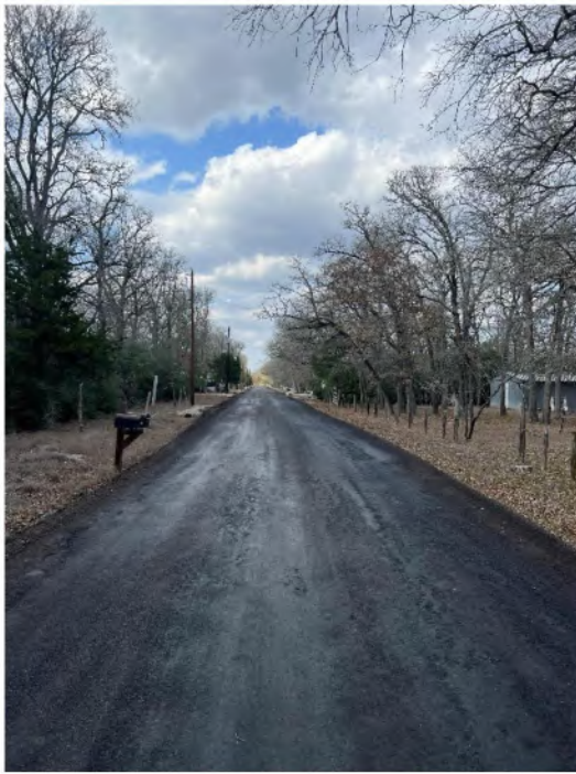
Figure 14 - Edgewater RAP Installation – 2/12/2026
