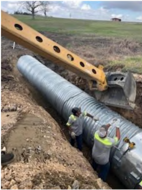
Figure 24 - Bosse Road Culvert Installation 3/5/2026
