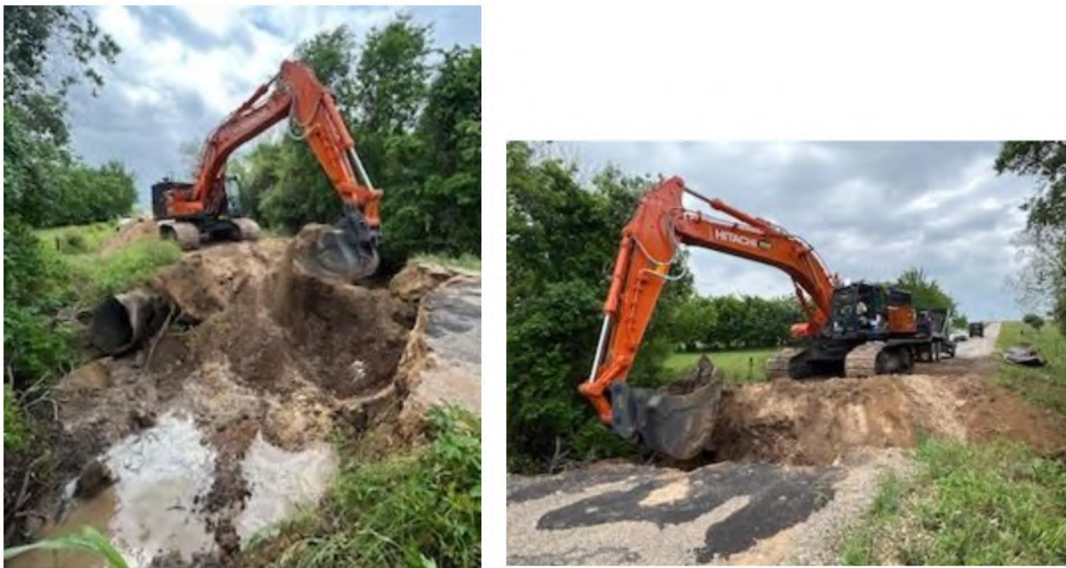
Figure 21 - Culvert replacement at Rocky Hill School Road 4/13/2026
